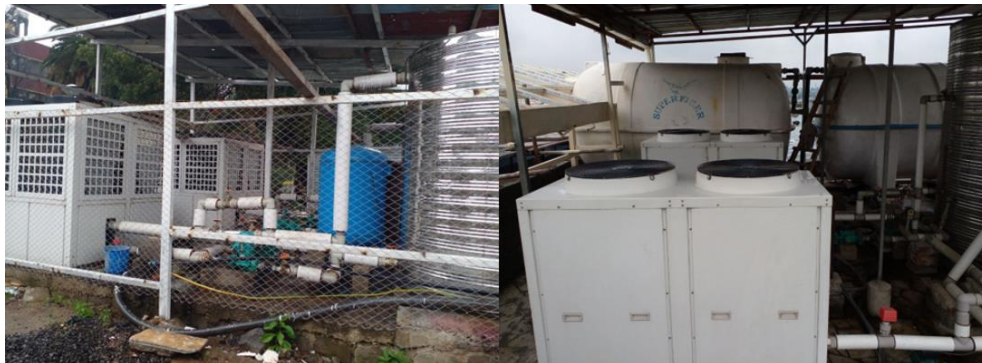
Figure 4-13: Some of centralized air to water HP system in hospital and health specialty centers
