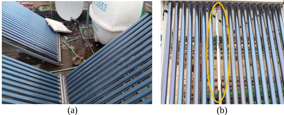
Figure 4-25: (a) Evacuated Tube SWHs installations and (b) broken glass tube
