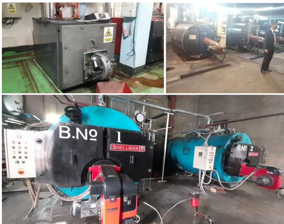
Figure 4-8: Some of centralized fossil fuel boilers in hotels
