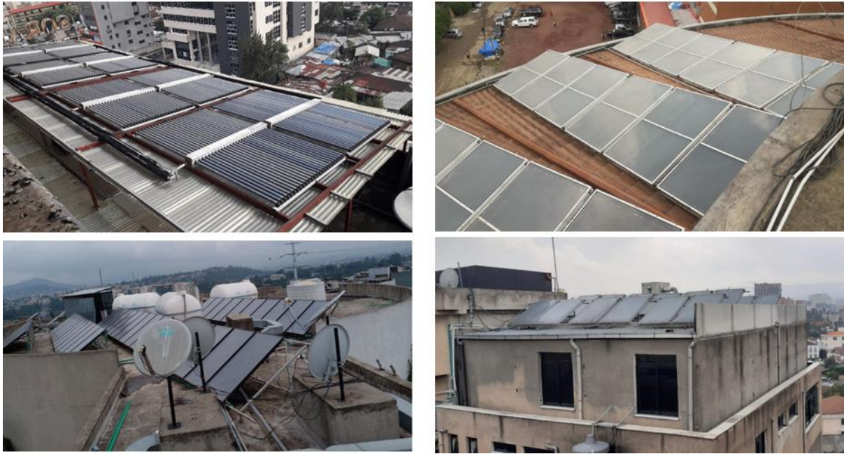
Figure 4-3: Collectors of some of centralized SWH systems in hotels
