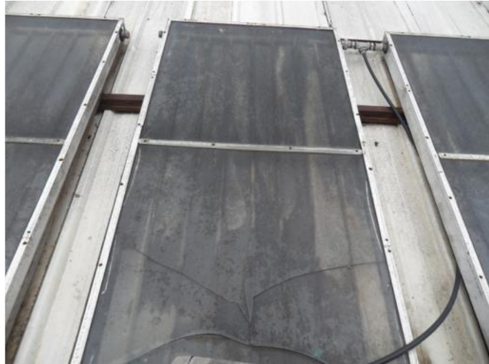
Figure 4-24: Broken glazing of flat plate collector type SWH
