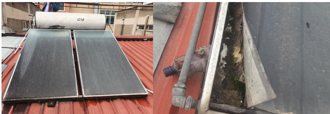
Figure 4-21: Flat plate collector type SWH under poor working condition
